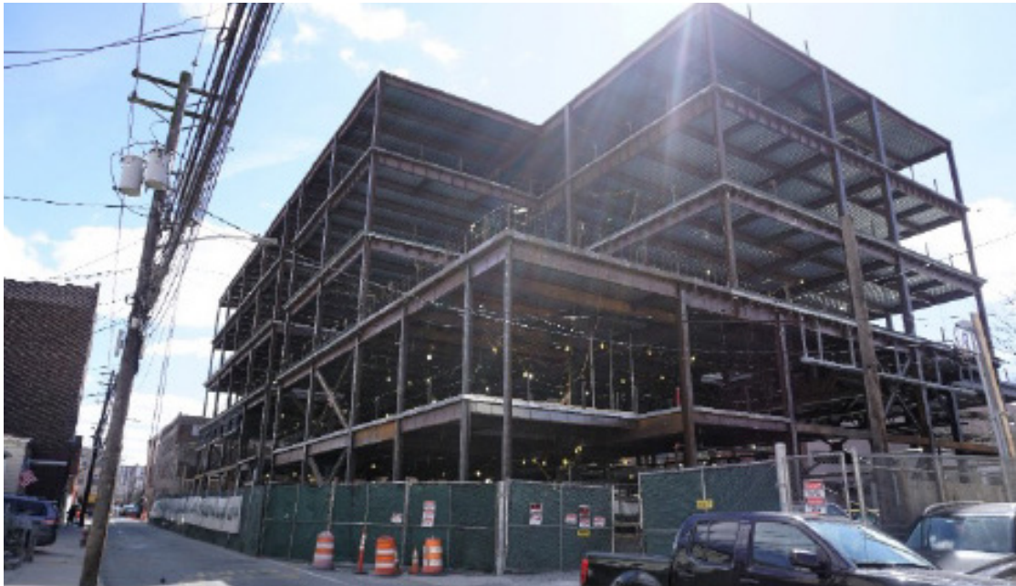
Picture above: Ongoing construction of the Union City Grade 7-9 Community School
